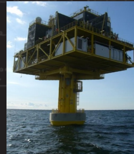
Offshore Wind Electric Service Platform (Substation)
